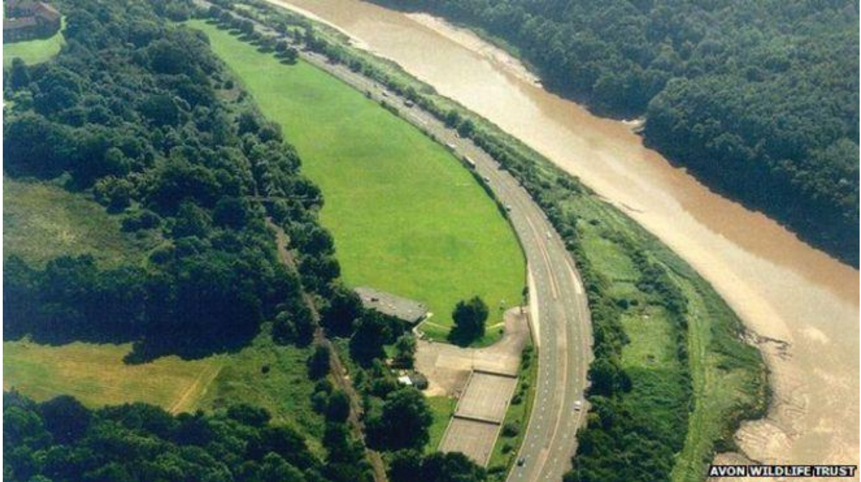
Image caption The site is alongside the Portway and the River Avon
